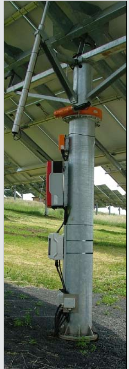
Connection to solar inverter with combination DC generator disconnect switch and DC surge arrester
